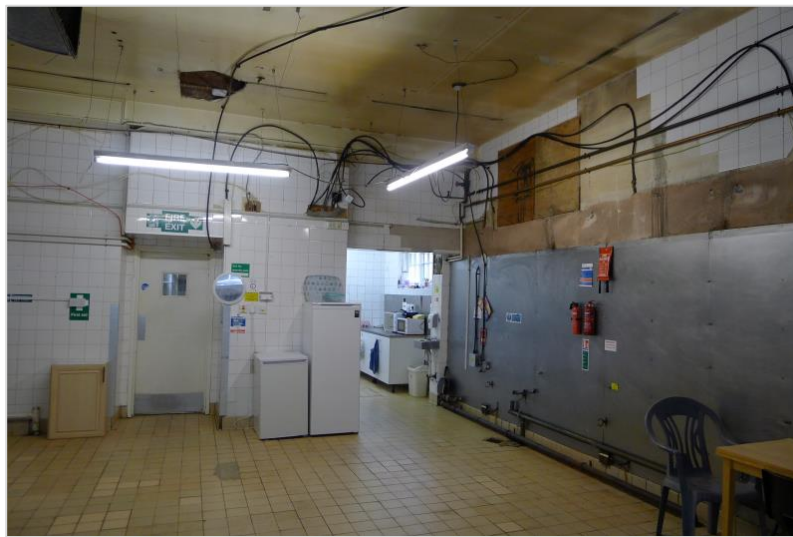
Figure 3.3: Existing Kitchen/Service Area
