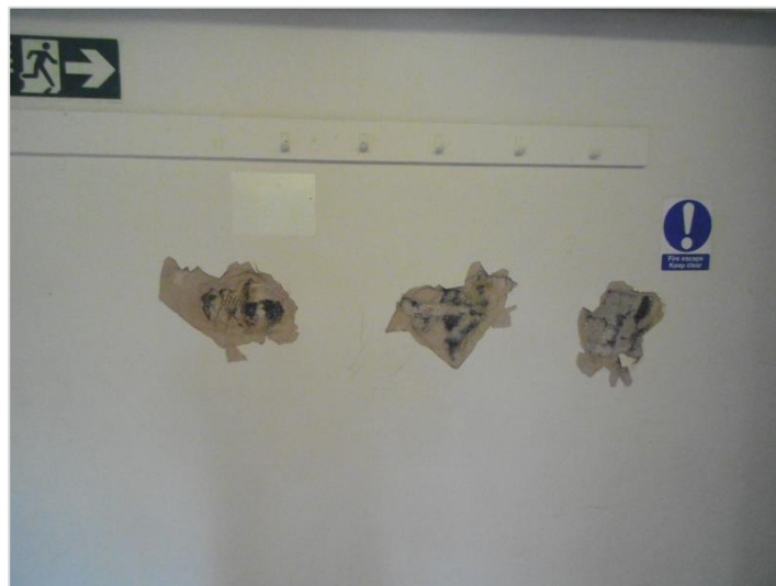
Figure 3.4: Modern Breezeblock Construction of Existing Wall
