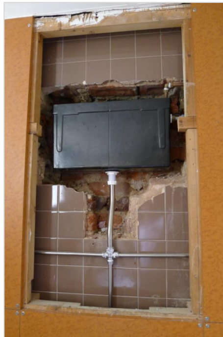
Figure 3.2: Existing Intervention into Proposed Location of Opening
