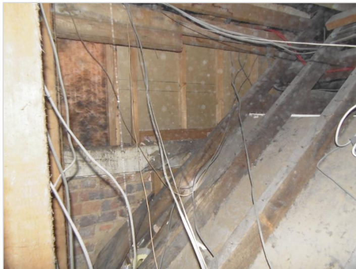
Figure 3.7: Obscured Roof Structure
